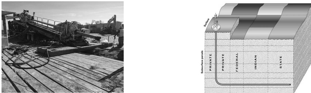
Figure 1 – Horizontal Borehole Drilling Rig and Directional Drilling Diagram. Wikipedia.
