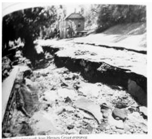
Figure 4 – Twelve Foot Deep Surface Failure North of Ottinger Hall and 400 feet north of proposed Well site, looking south, June 9, 1983. Salt Tribune. 1983. Spirit of Survival: Utah Floods of 1983.
