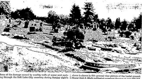
Some of the damage caused by rushing walls of water and mud during through the Salt Lake City cemetery during Sunday night's storm is shown in this general view picture of the burial ground. Mayor Earl A. Glade estimated cemetery damage at over $50,000.
